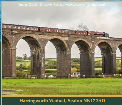
Harringworth Viaduct, Seaton NN17 3AD
